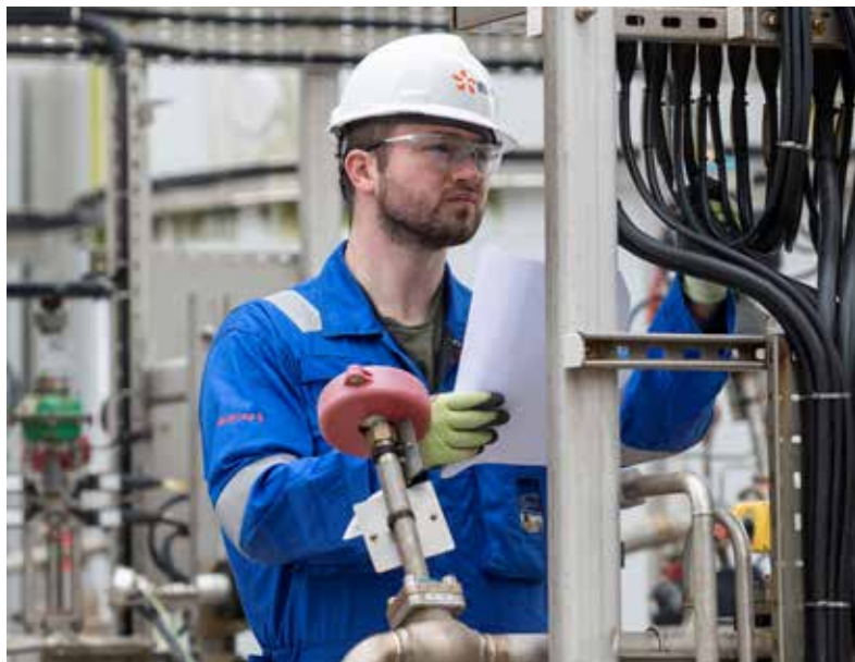
Intervention de maintenance Hinkley Point B
