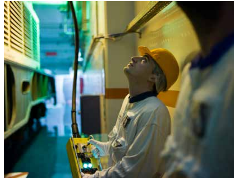
Manutention château combustible Cruas
